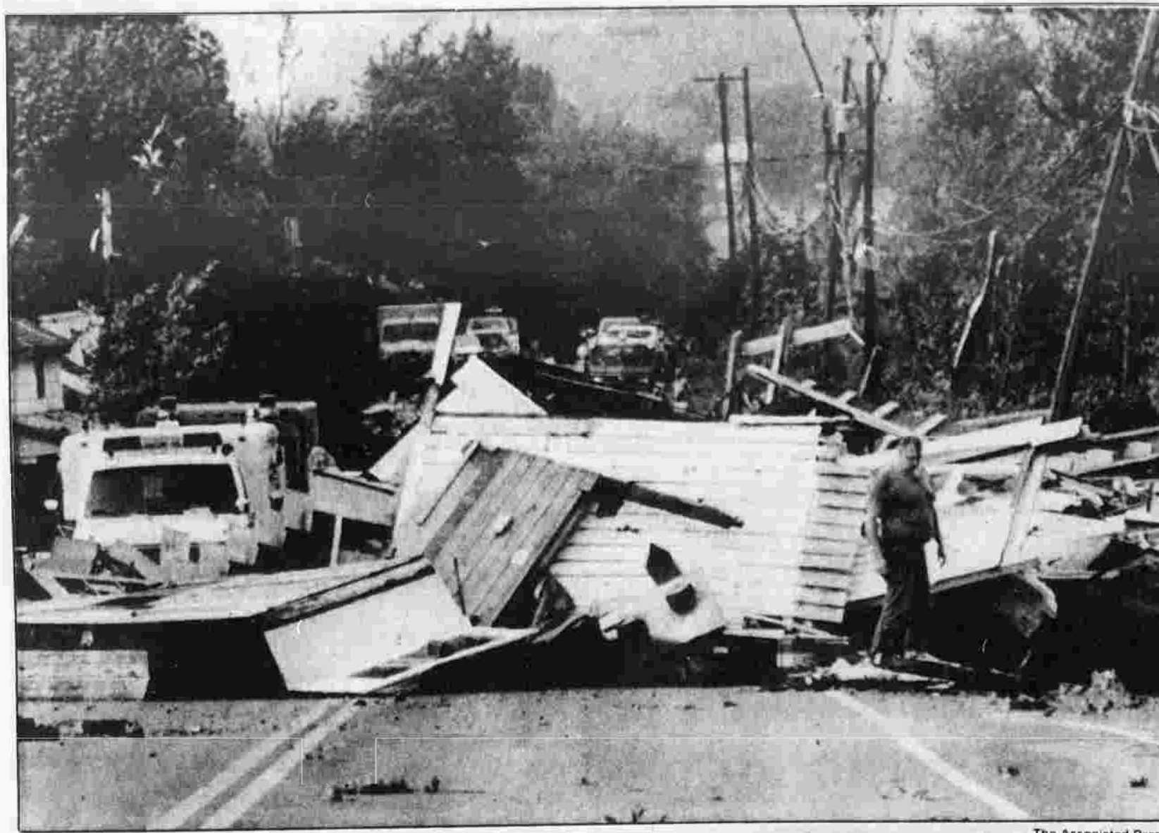
Bob Brazile inspects his house which the storm blew onto Route 7 in Howes Cave, N.Y., Monday afternoon. At least two people were killed, dozens injured and hundreds left homeless by the storm.
